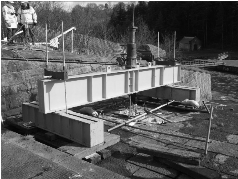
Figure 4. Equipment for load testing of channel invert blocks
